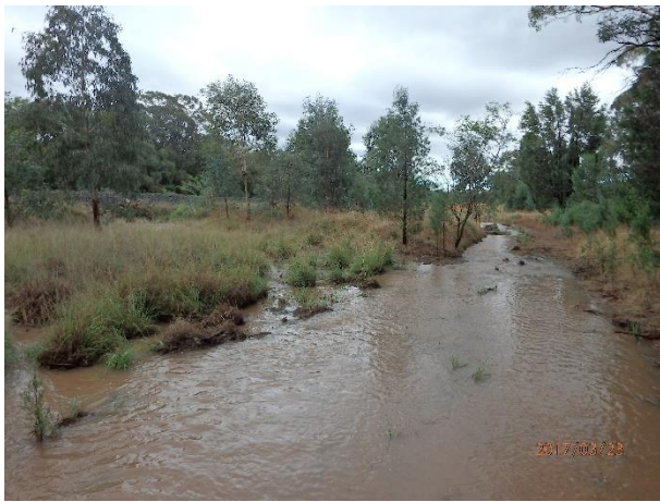
Plate C1.19 – Flooding on the unnamed lane that runs parallel to the railway to its south (Photo taken at 09:14 hours)
