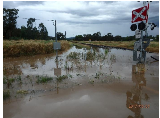
Plate C1.6 – Looking west along southern (downstream) side of railway from Flagstone Street ( Photo taken at 08:21 hours )
