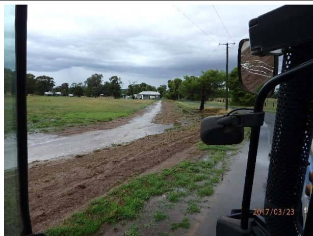
Plate C1.8 – Looking south along channel on eastern side of Flagstone Street (Photo taken at 08:38 hours)
