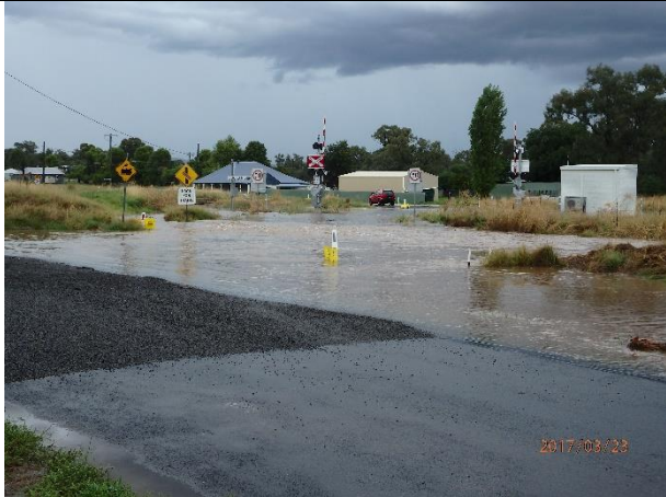
Plate C1.1 - Looking south at Flagstone Street level crossing of the railway ( Photo taken at 08:17 hours )
