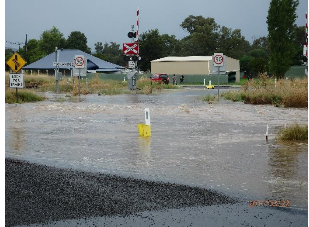
Plate C1.2 - Looking south at Flagstone Street level crossing of the railway ( Photo taken at 08:17 hours )
